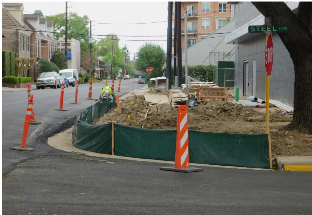
11. Sidewalks being readied for concrete.
