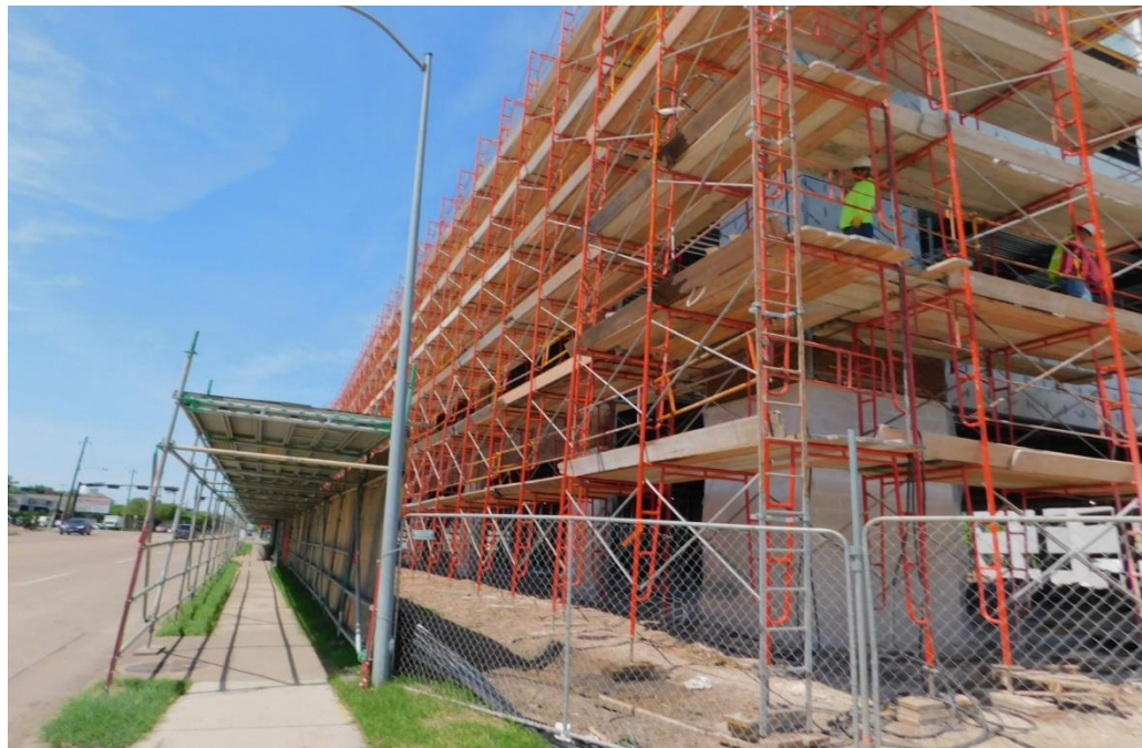
5. Brick work has begun on front of building.
