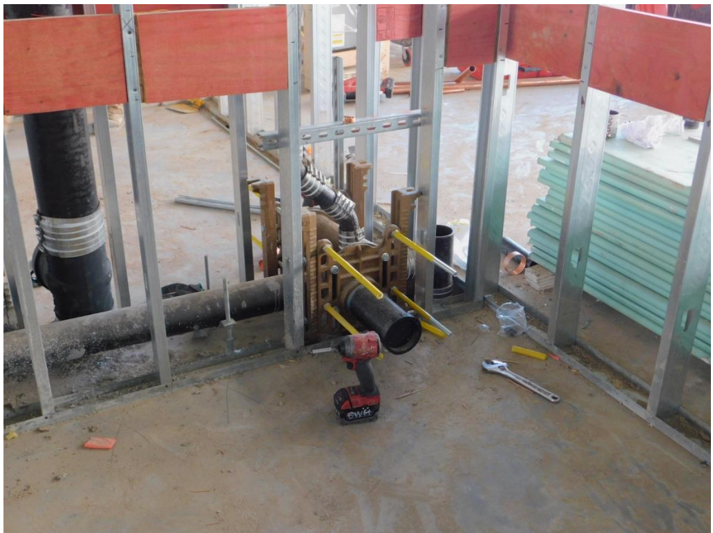
3. Electrical and plumbing roughed in on each floor.
